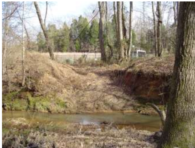
Embankment cut on Clems Branch. Possible historical road crossing. View south over creek to campground in the distance.
