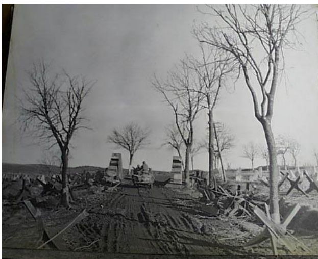
Passageway through Siegfried Line of land mines, tank traps, and dragon teeth
